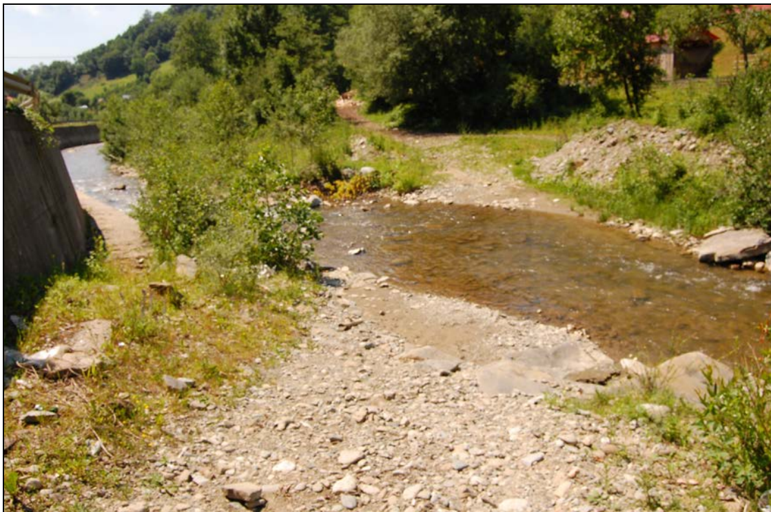
Figure 7: Frumuşeaua River concrete riverbank/completely modified and road in the riverbed.
